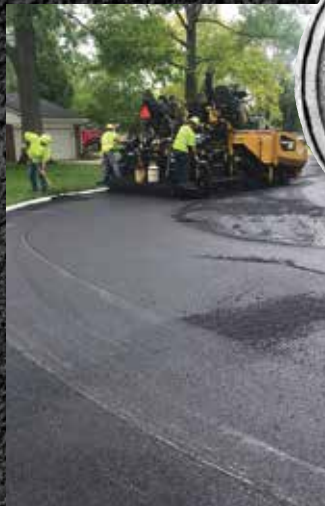
Resurfacing work on Glenburn Drive
