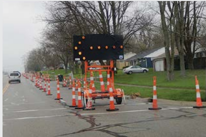
Alex-Bell Road undergoes improvements.
