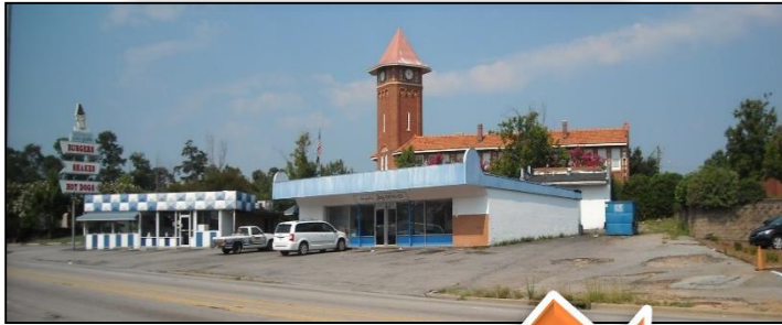
Before the improvements
