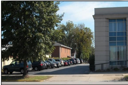
Before the improvements
