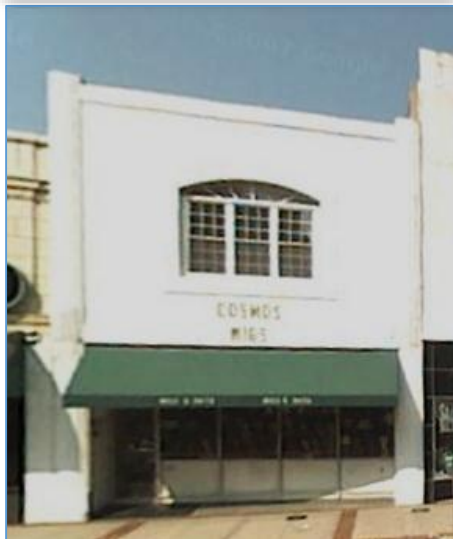
Before the improvements
