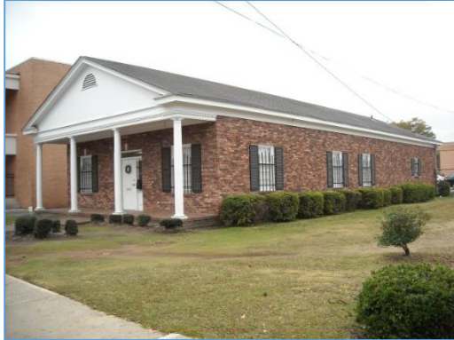
Before the improvements
