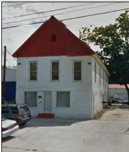
Before the improvements
