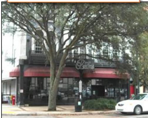
Before the improvements
