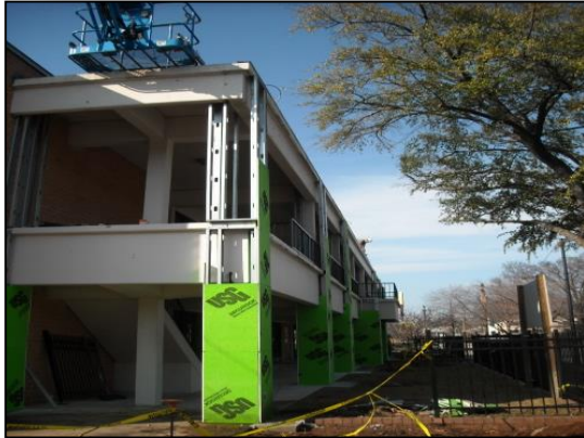
Before the improvements
