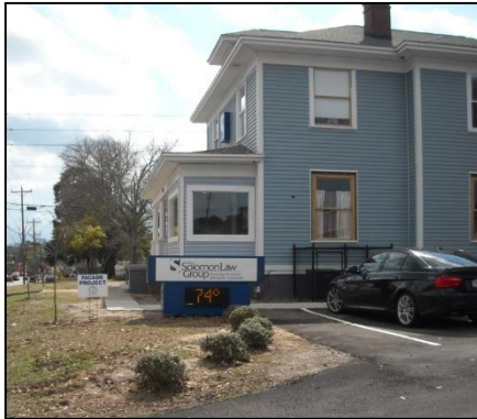
Before the improvements
