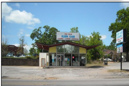
Before the improvements
