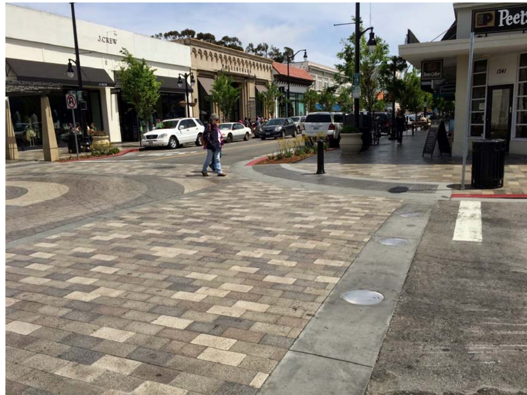
Pavers or similar materials should be used to both accent the site and provide clearly defined pedestrian crossings .
