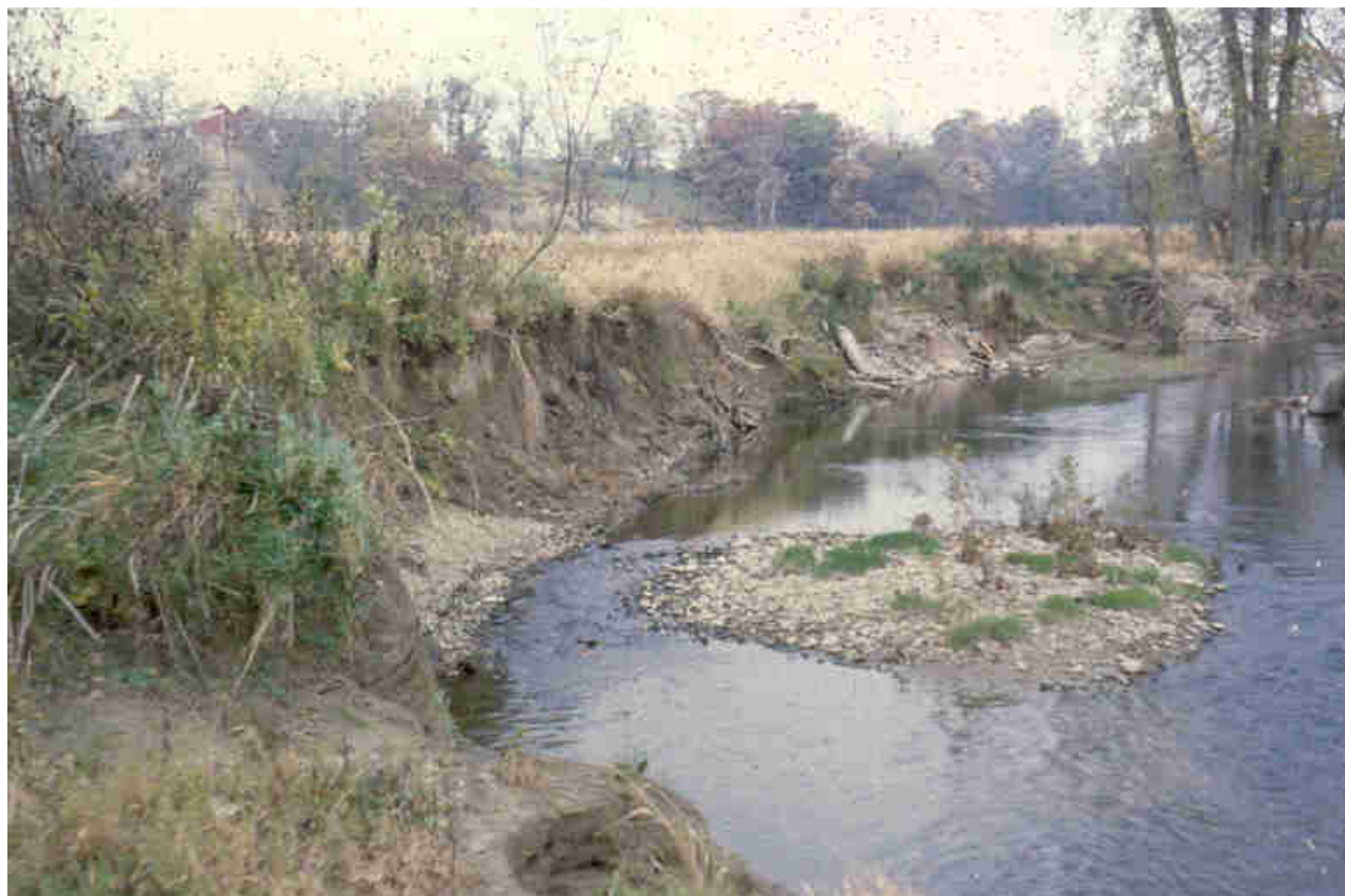
Figure 24. This area of Ross silt loam along Twin Creek is susceptible to stream bank erosion.
