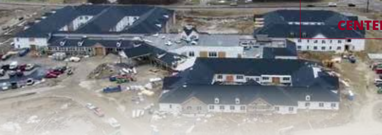
Aerial view of Randall Residence, estimated to be completed in May
